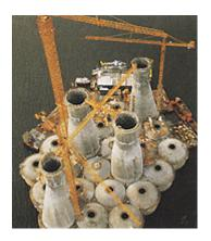
The 24 cells and 4 shafts referred to above are shown to the left while at the sea surface. The cells are 12m in diameter. The cell wall failure was traced to a tricell, a triangular concrete frame placed where the cells meet, as indicated in the diagram below. To the right of the diagram is pictured a portion of tricell undergoing failure testing.
